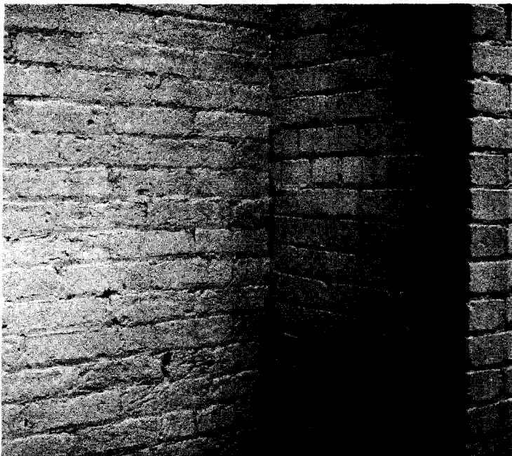
1882 Hand-moulded brick on the left used in the construction of the Hayt-Wientge Mansion and machine pressed brick on the right utilized in an 1899 addition.
