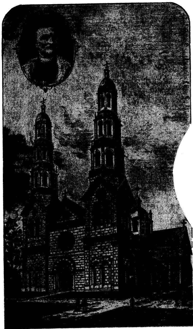
The Cathedral of St. Francis was originally designed with steeples rising to a height of 160 feet, side chapels replacing the Chapels of La Conquistadora and San Jose and a large dome above the transept. The plans, however, were never completely executed. Reprinted from: William G. Ritch, AZTLAN. Boston, 1885.
