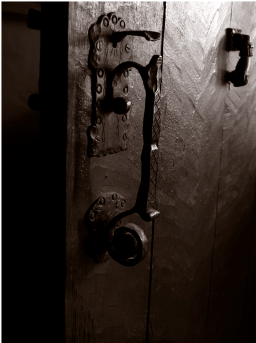
The front door of the Henderson House is hand-adzed with custom hand-made hardware. Photo © Steve Northup.
