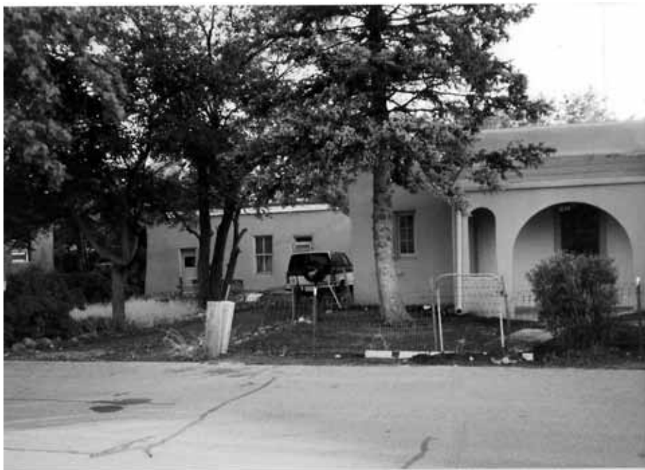
Figure 7: House before 1989 upgrade project, courtesy Joseph Valdes
