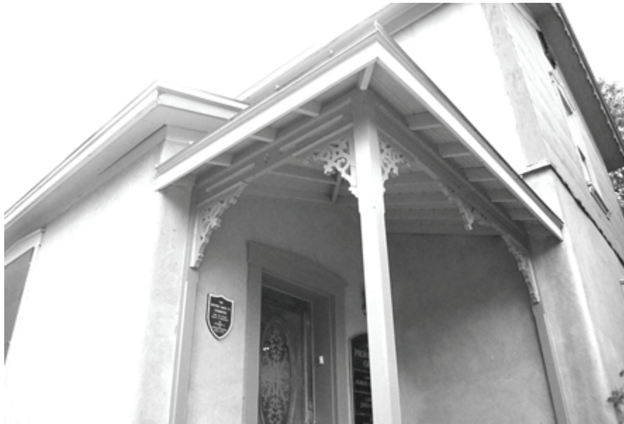
Delicate post brackets with centered pediment of the front porch.
