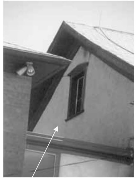
Original window frame on main building. © Corinne Sze 1999
