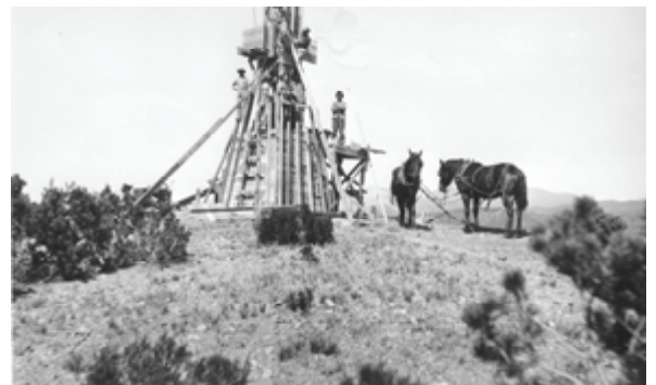
Construction of the Cross, 1919-1920. Courtesy Palace of the Governors (MNM/CDA)#57998.
