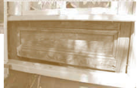
Work on the Oliver P. Hovey house at 136 Grant Avenue this year included re-roofing the bay window on the south side. Some plaster repair was required including recreation of the faux bricks finish. Below, the original raised wood panels were uncovered and restored as they appear in the circa 1890 photo on the left.
