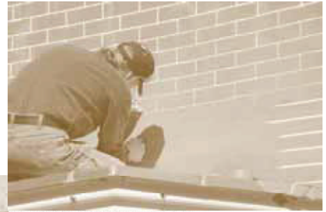
Work on the Oliver P. Hovey house at 136 Grant Avenue this year included re-roofing the bay window on the south side. Some plaster repair was required including recreation of the faux bricks finish. Below, the original raised wood panels were uncovered and restored as they appear in the circa 1890 photo on the left.
